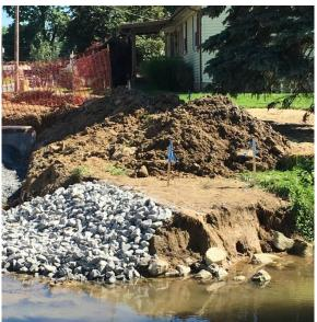
Do cover stockpiles or implement sediment control devices such as silt fence—especially when rain is forecasted—so rain does not carry sediment off into storm drains or directly discharge to streams. Soil should not be stockpiled on the street either. Downstream inlet protection may need to be implemented for large stockpiles for "back-stop" protection.
