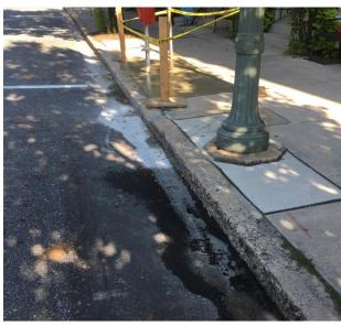
Do implement temporary protection measures for inlets that may be off site or can receive drainage from the work area. This may entail temporary sealing off an inlet for saw-cutting work and cleaning up the residue after work is complete. Please note: inlets should not remain sealed off if it is raining, and residue needs to be cleaned up before removing controls.
