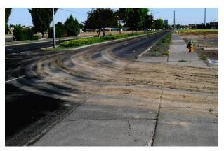
**Do** sweep up and/or remove tracked sediment. This should be done at the end of every working day, after higher volume of traffic has left the site, and/or before forecasted rain events. Consider upgraded temporary construction entrances that deploy rumble plates (corrugated steel panels) or "tire racks" that collects sediment from washing off tires if tracking sediment is consistent issue.
