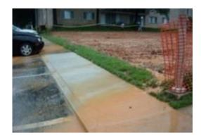
Do implement temporary soil stabilization controls if permanent stabilization cannot be installed yet—especially prior to forecasted rain to reduce the potential of sediment-laden runoff entering the MS4 or streams. Soil stabilization is an erosion control practice. Erosion and sediment control devices should be implemented in conjunction with each other—not independent of each other.
