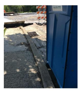
Do place temporary toilets greater than 50 feet from storm sewer inlets and/or waterways. Ideally, temporary toilets are placed at a low point away from inlets where any spills or overflows can be contained by the topography. Consider implementing spill control berms (e.g. spill dike) or a portable toilet containment pan to contain a spill if conditions do not allow placement greater than 50 feet from or in drainage patterns to a storm sewer inlet.
