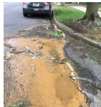
Illicit Discharge (sediment-laden runoff from utility boring) to an MS4 inlet.
