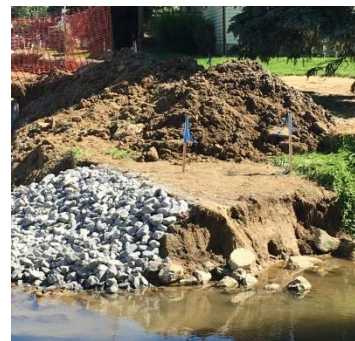
Unprotected stockpile and exposed soils on an active construction site that should have erosion and sediment controls in place.
